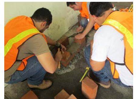
Photo 2 Construction of prism specimens (UES)
