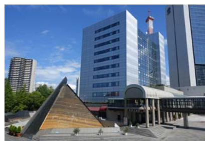
Photo 1 Kobe International Conference Center
